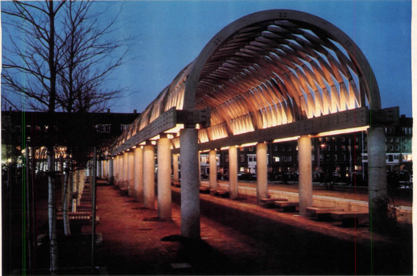
Laminated wood trellis at Boston Waterfront Park, Boston, Mass. Wood structure supplied and assembled by Unadilla Laminated Products, Unadilla, N.Y. Architect, civil engineer, landscape architect: Sasaki Associates, Inc., Watertown, Mass.
