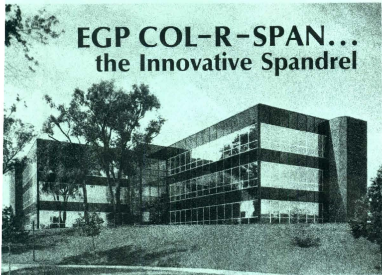
Crowe Chizek Bldg., South Bend, IN; Architect - Cole Assocs., Inc.; Glazing Contr. - Interstate Glass; EGP COL-R-SPAN (black) & EGP COOL-VIEW reflective (clear with chrome coating)
