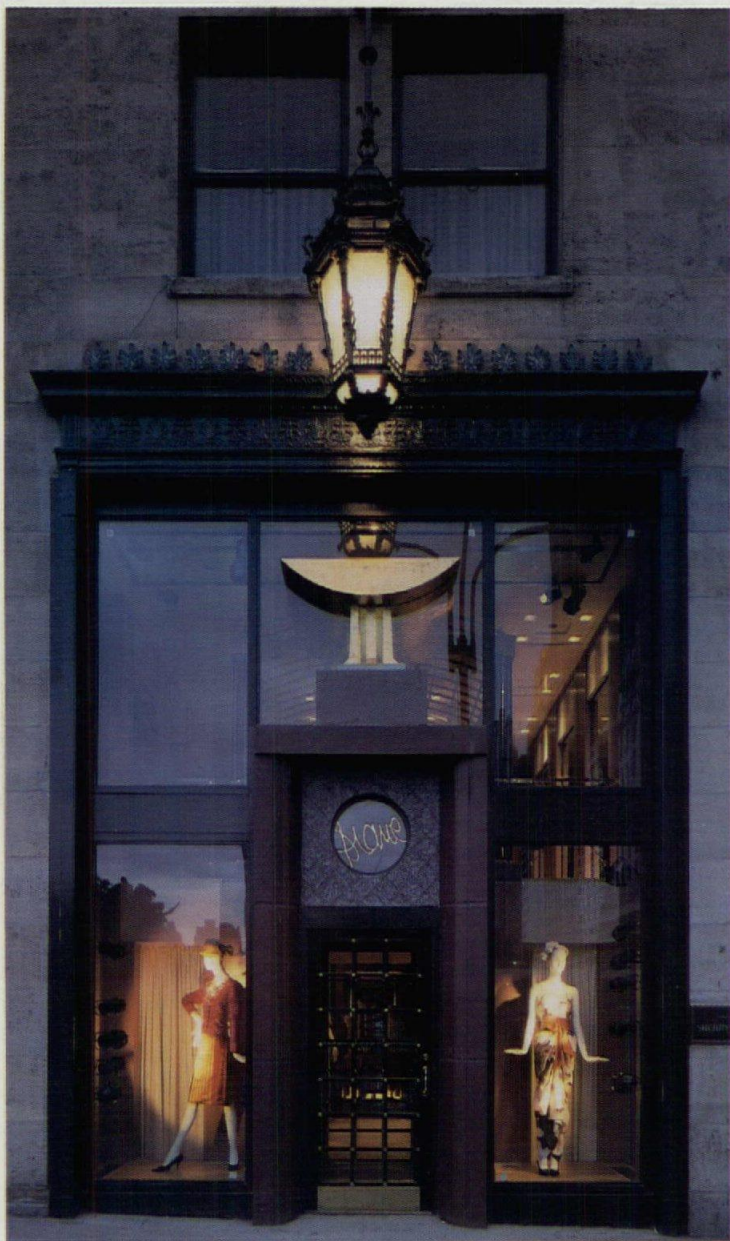
Diane Von Furstenberg Boutique New York City Architect: Michael Graves Architect 341 Nassau Street Princeton, New Jersey 08540 Michael Graves, principal; Theodore Brown, associate-in-charge; Robert Marino, job captain; Anita Rosskam and Tom Rowe, assistants Engineers: Desimone & Chaplin, (structural); Kalen & Lemelson, (mechanical/electrical) General contractor: Pavarini Construction Company Photographer: ©Peter Aaron/ESTO
