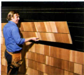
Install 8-feet of shingles in a shake.
