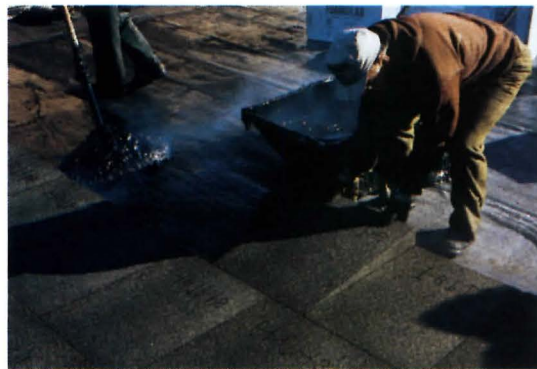
A Tapered FOAMGLAS® Roof Insulation System was specified for the re-roofing of the library.
