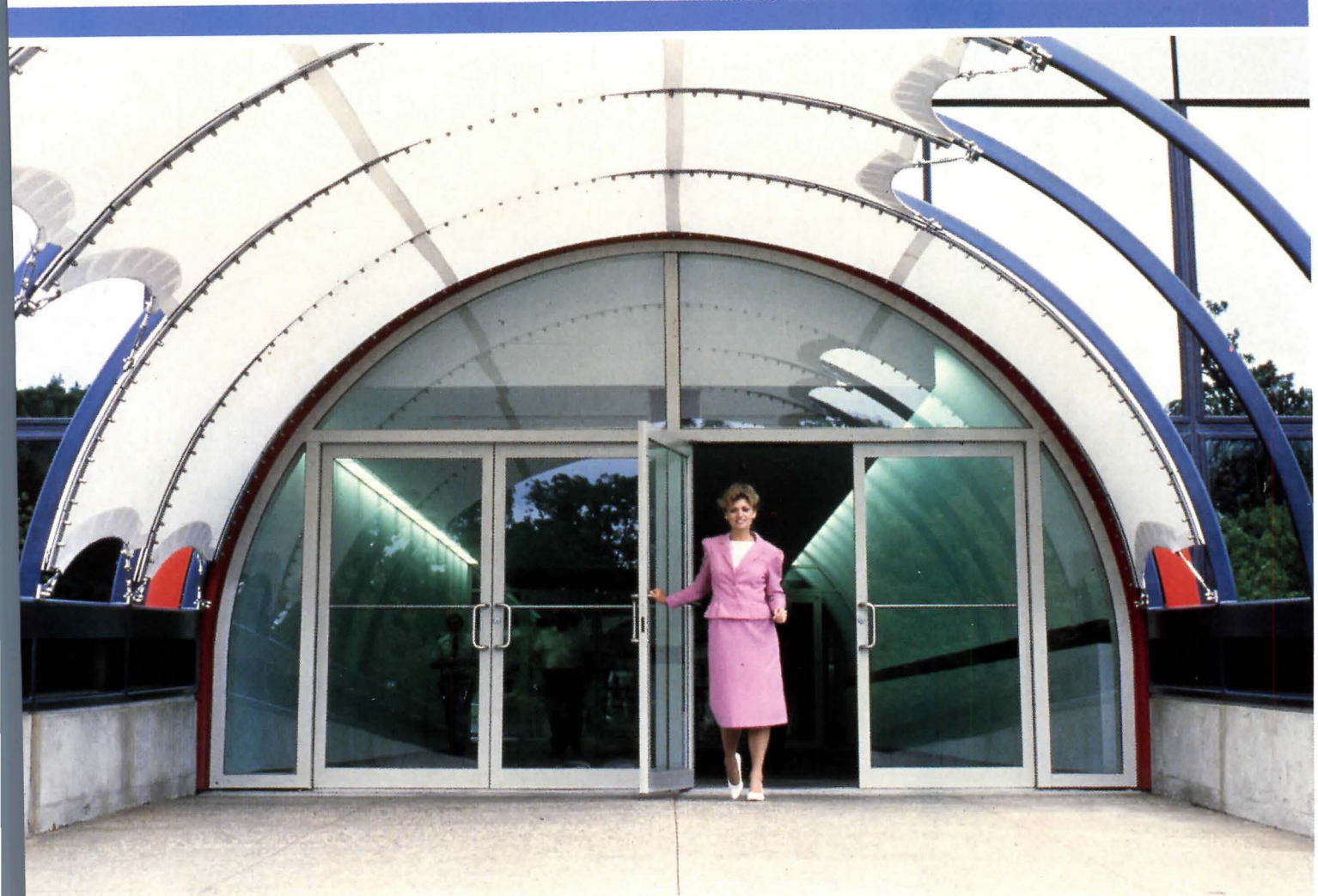
Illister, Inc., Corporate Headquarters, Libertyville, IL; Holabird & Root, Architects, Chicago, IL
