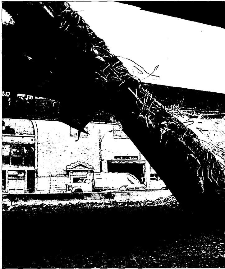
The gradual deterioration and ultimate collapse of the West Side Highway in Manhattan led to the initial proposals for Westway.
