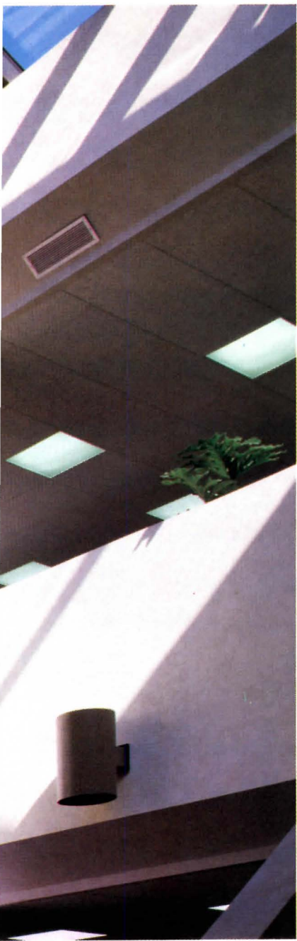
STANDARD GRID with its wide 1 3/16" exposed face provides for a ceiling design that is coarse by today's standards. Shown above with standard square-edge lay-in panels.
