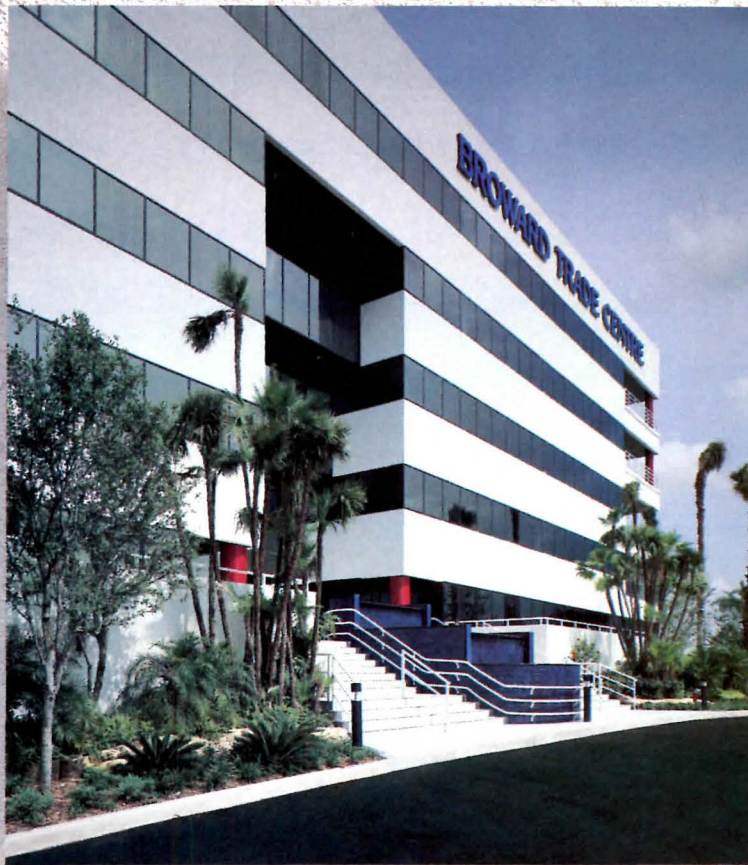
Broward Trade Center Fort Lauderdale, FL. Certified Applicator: RAMCO, Inc. General Contractor: Knight Enterprises
