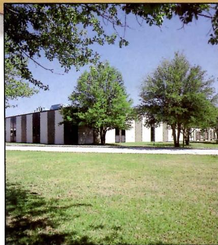
Bill Knapp's Restaurant Distribution Facility
