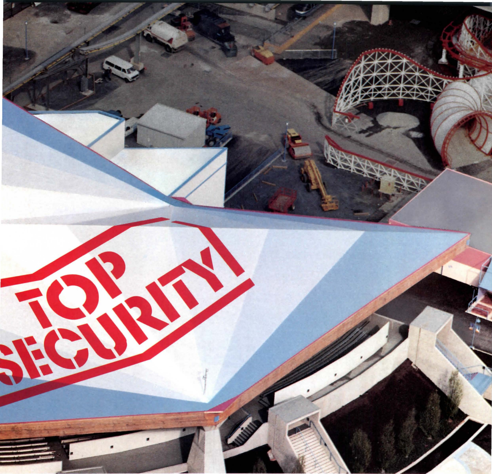
Single-Ply Roofing Roofing Manufacturer: Dunlop Construction Products, Inc., Mississauga, Ontario, Canada; Dunseal Hypalon™ H301 System
