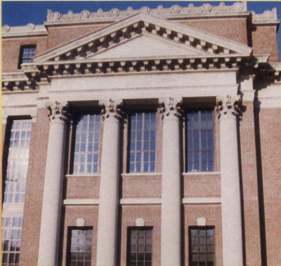
Widener Library, Harvard University. Original casement, awning and fixed windows were reproduced. Precise physical dimensions and projections for all profiles were maintained within 1/32 of an inch as specified.
