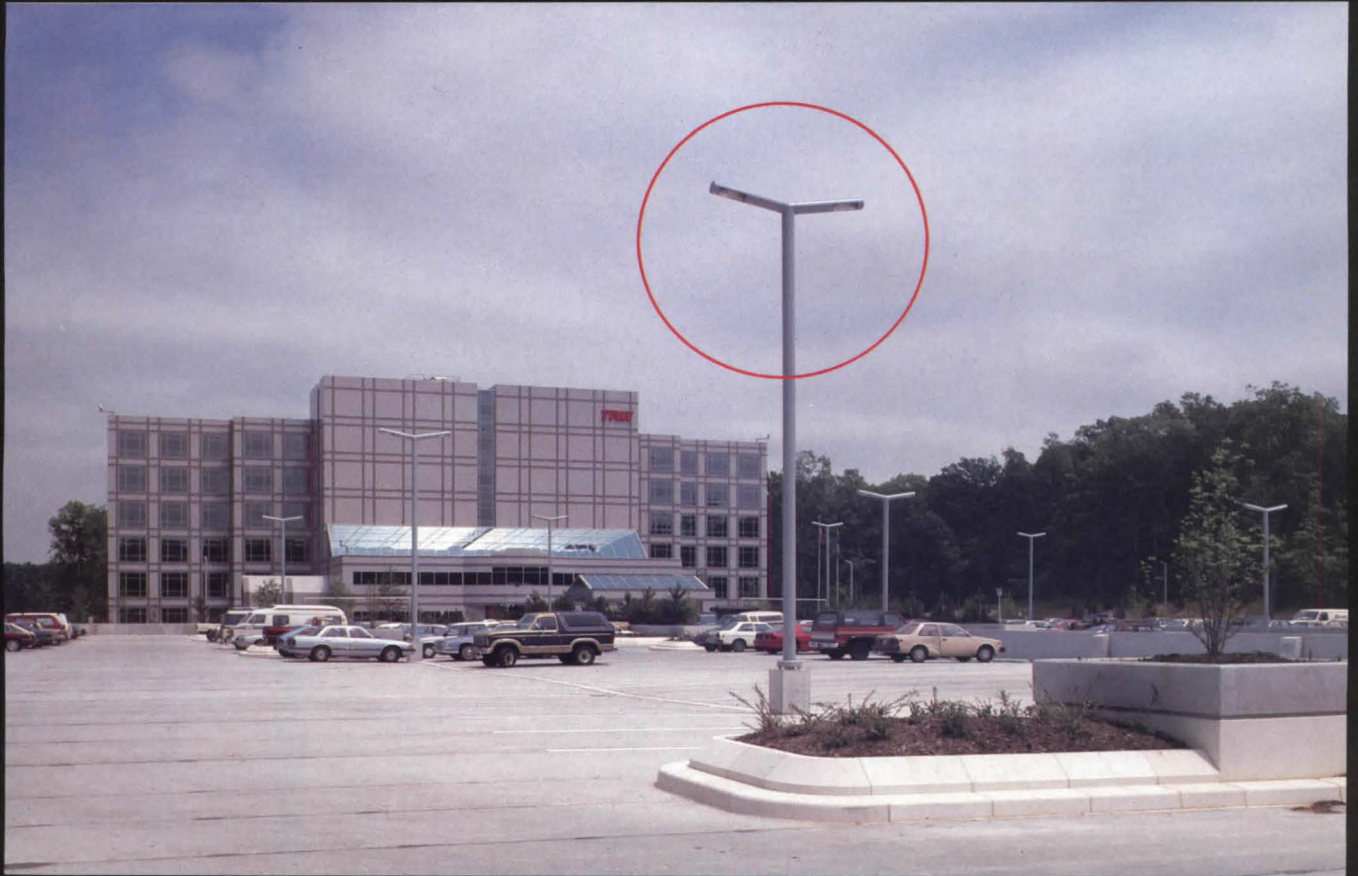
TRW Building, Fairfax County, Virginia
