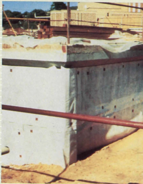
Contech STRIPDRAIN 75 drains more water than a 14'-thick sand or 17"-thick gravel drain.
