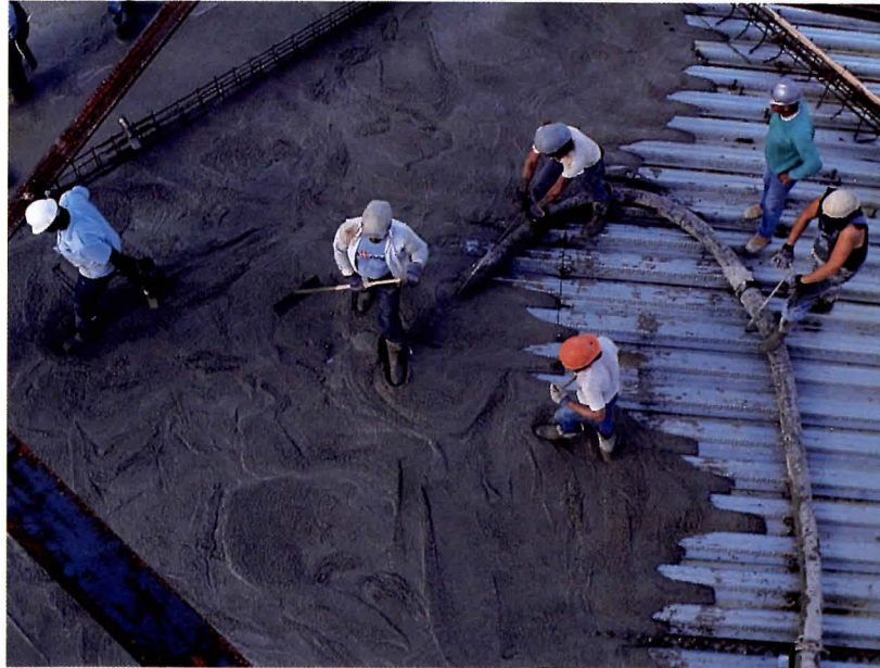
Installing Vulcraft composite deck is faster and more economical than poured-in-place concrete.
