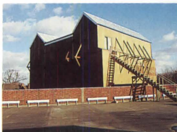
Exterior of full-scale mockup
