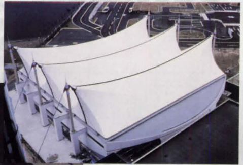
Point-hung tensioned membrane structure at Toyohashi.
