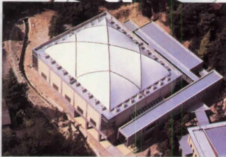
Translucent membrane roof brings daylight to college gymnasium at Hiroshima.
