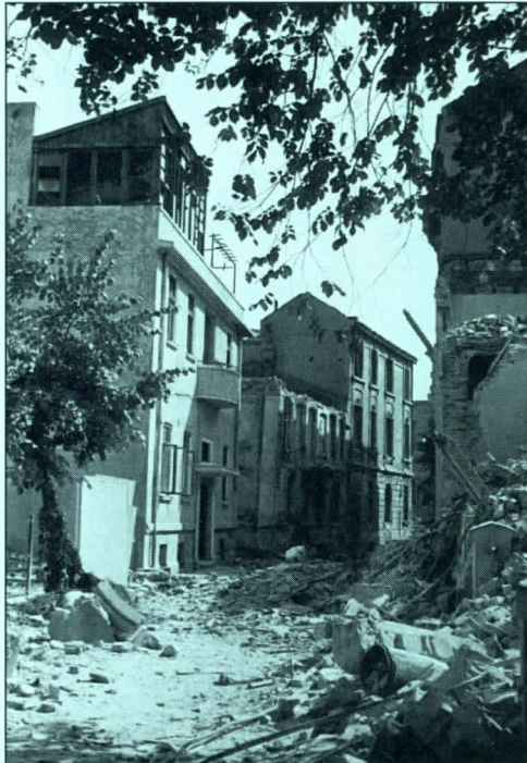
A neighborhood in Bucharest is ripped by demolition in 1985.
