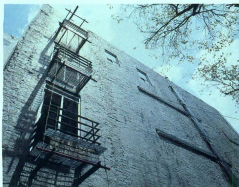
Above: The exposed structure, underlined by suspended raceways, sets off such sleek forms as the main showroom's granite and metal counter and galvanized-metal screen. Below: The rear facade is marked by a row of balconies and a "tree" of conduit that feeds interior electrical grids.
