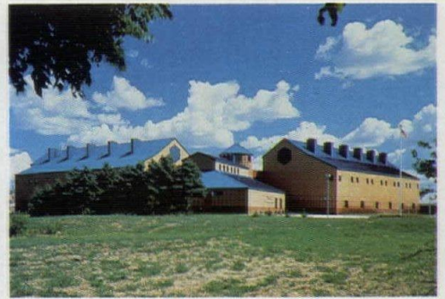
The crop science complex heads a row of existing greenhouses (site plan). Electron microscopy is performed in the skewed structure (plan). Moving counterclockwise are sunflower research; seed cleaning, drying and storage; existing greenhouse; sugar, grain, and beet research.
