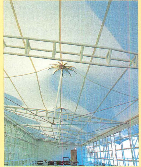
Fabric roofs cover the atrium and a gallery at the Imagination Building.
