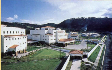
U. S. Embassy, San Salvador, CRSS Sirrione International, Architects.
