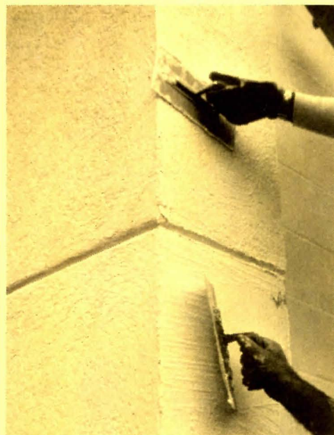
Installation involves a trowel-on technique. Photo, courtesy of Thoro System Products.
