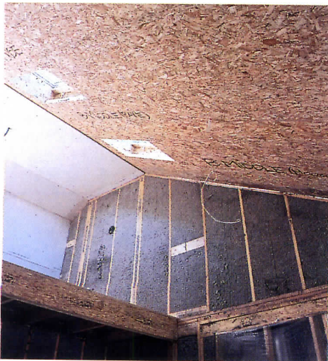
IBACOS's roof system mockup
