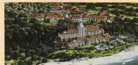
Nanhai Oil Building in Shenzhen, China, by the Nadel Partnership and Nanhai Design Institute (top), and the Bali Nikko resort by WATG and Airmas Asri (above).
