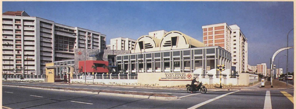
As areas outside Singapore's central core grow, facilities like the Tampines Community Center (below), designed by William Lim Associates, are needed.
