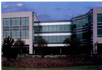
B.C. Hydro Edmonds Centre; Vancouver, B.C.: EverGreen Glass outboard and Energy Advantage Low-E Glass inboard; new construction project.
