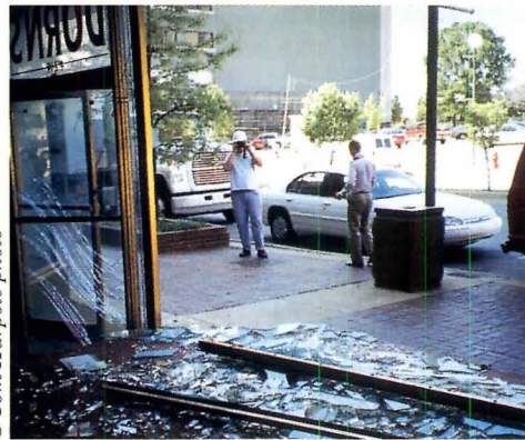
The Oklahoma City bomb blast showed the different behavior of annealed storefront glass and laminated glass (held in frame).
