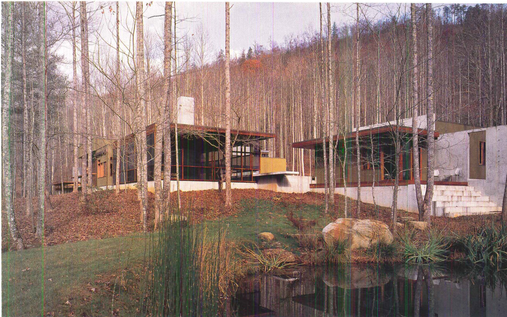
Moving around the house: the entry court with the main house and screened porch (below), the guest house seen from behind (above), and the south elevation (opposite, top and bottom).
