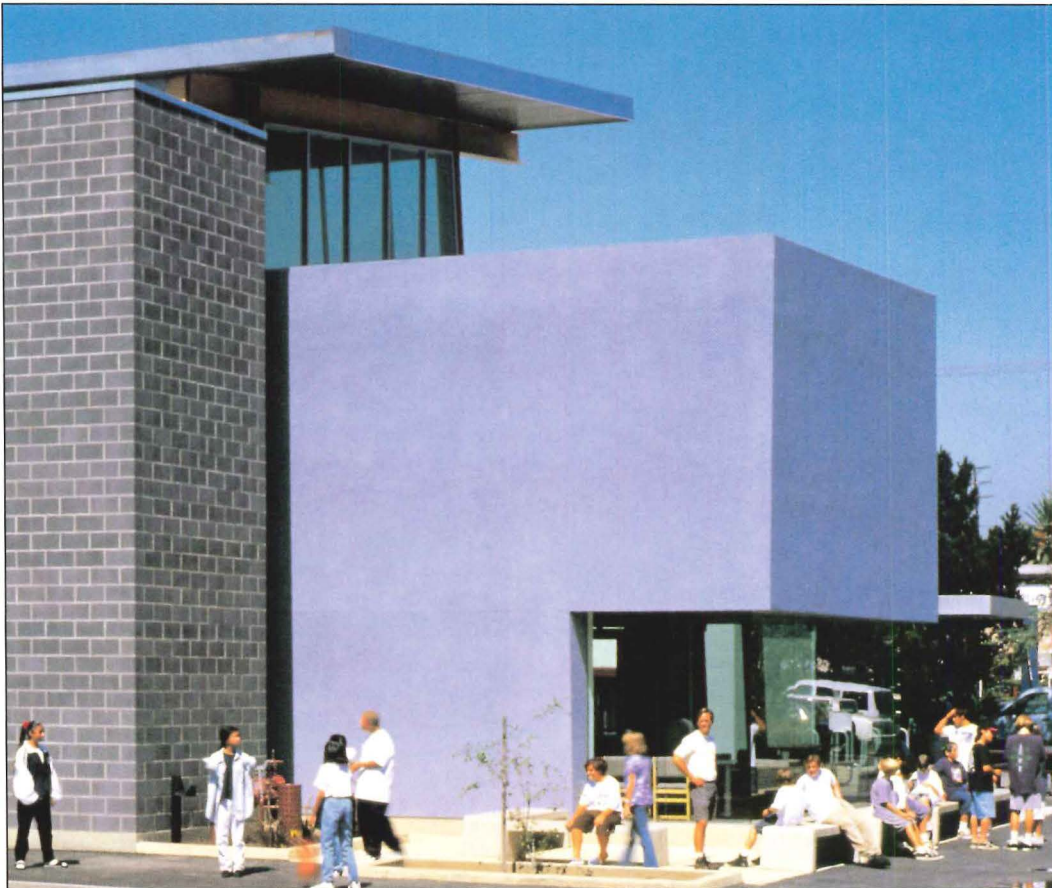
Left: An architectural "wedge" rises out of a campus alley to house the Paul Cummins Library. Construction of this project included approximately 5,000 square feet of concrete masonry.
