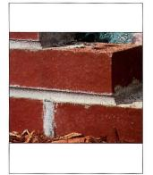
are inexpensive and easily installed in weep holes to insure masonry cavity walls breath, drain and dry quickly. Made from 100% recycled polyester with a 90% open mesh in 2.5" x 4" x .5, they are available in white, tan, almond, gray, and brown. Weep Vents add to the beauty of the wall by duplicating the texture and color of mortar. thus eliminating open holes and dark shadows while restricting entry to insects. Call (800) 664-6638 for more information.
