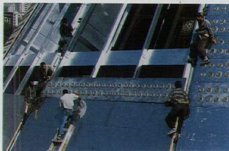
The main facade of the 250,000-square-foot International Conference Center in Teheran (above). Local laborers work on the dome, whose panels were fitted with 40,000 glass cylinders (left).
