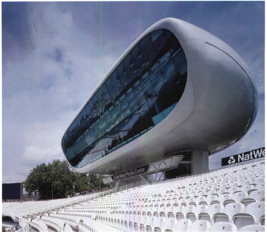
The media center had to be prefabricated in shipyards and cost over $9 million to construct and install.
