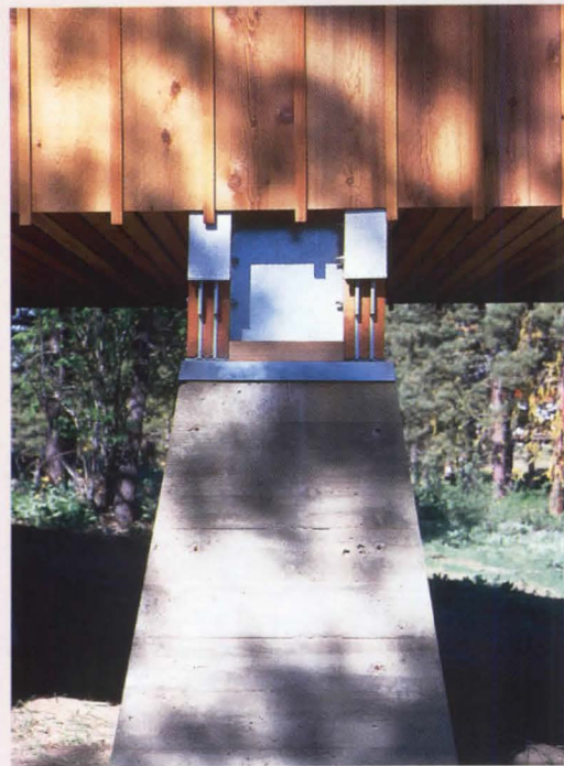
Detail 4: foundation section
