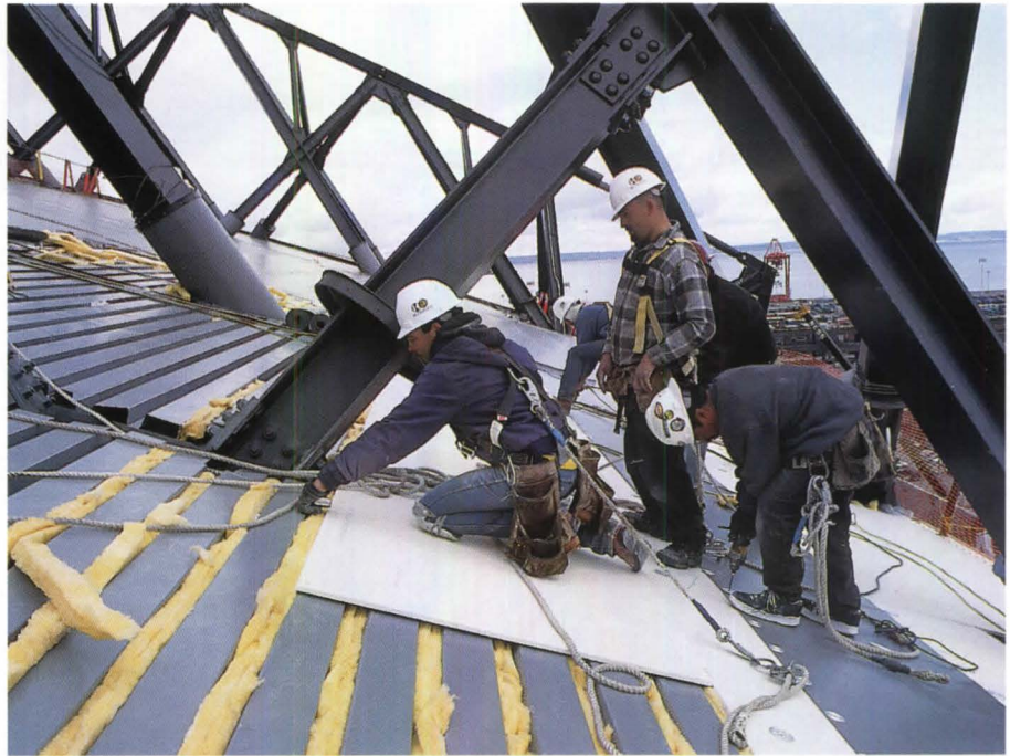
Working 200 feet in the air, roofers applied PVC to Safeco Field's roof.
