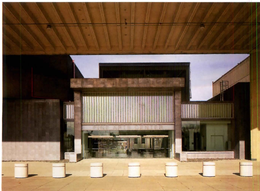
Two types of glass offer differing levels of transparency to direct the viewer's gaze through the building (above and below). Colored lights animate the south elevation at night (below right).
