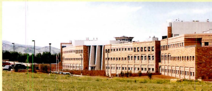
Project: David Skaggs Research Center, National Oceanic & Atmospheric Association, Boulder, Colo.
