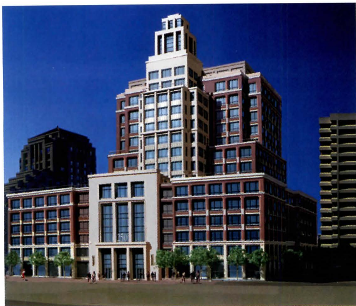
The Gap Embarcadero (above), by Robert A. M. Stern Architects and Gensler, includes slotted-web connections and a seismic core (below).
