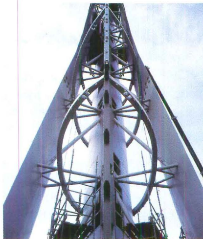
Two airfoils flank a central tower shaft.
