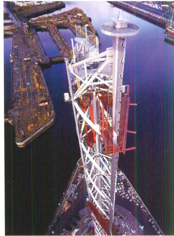
The Glasgow Science Center tower rises to 462 feet, with a viewing cabin at the 330-foot mark.
