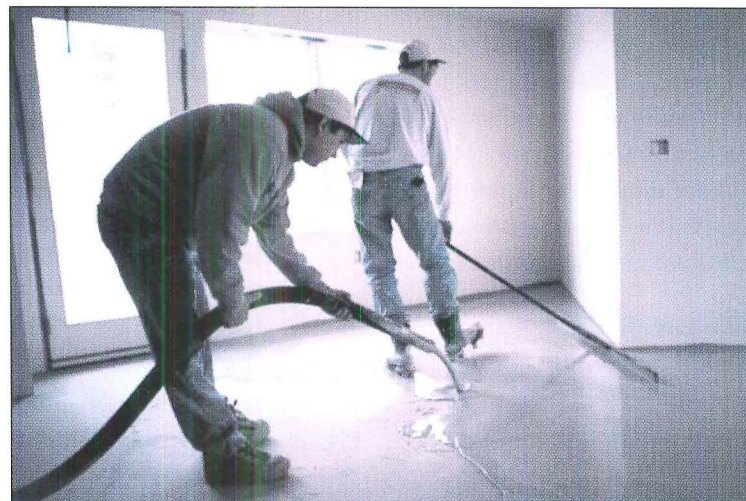
Due to its light weight and excellent sound control properties, gypsum concrete underlayment is the leading underlayment choice for multifamily construction.
