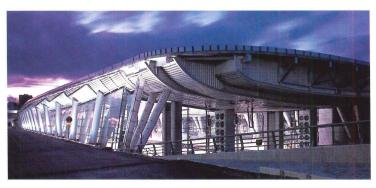
The two rows of splayed, paired columns at platform level are beefy enough to hold up the later addition of commercial space as well as massive trusses largely concealed within the metal cladding of the hull-shaped ticketing level. By spanning the full width of tracks, the trusses leave the platforms column free.
