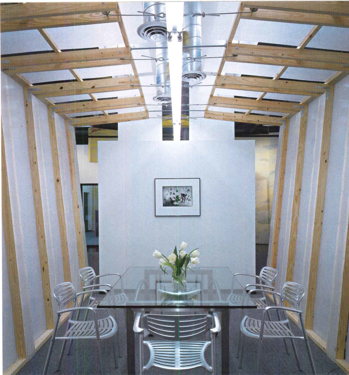
The conference room's canted walls are polycarbonate panels set within a frame of pine studs (left). The cabled canopy leaves HVAC ducts exposed. There are few right angles and many apertures for peering into adjacent rooms (below left).
