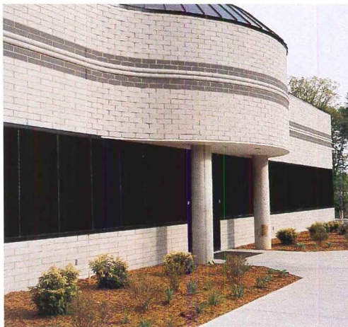
Coca-Cola Bottling Company of Northern New England, Inc., Londerry, NH Architect of Record/Engineer: Stahlman Engineering Corporation, New London, NH Accent Panels: 3 5/8" x 23 5/8" x 3 5/8", #M115, #M1428 Finish: Tudor®
