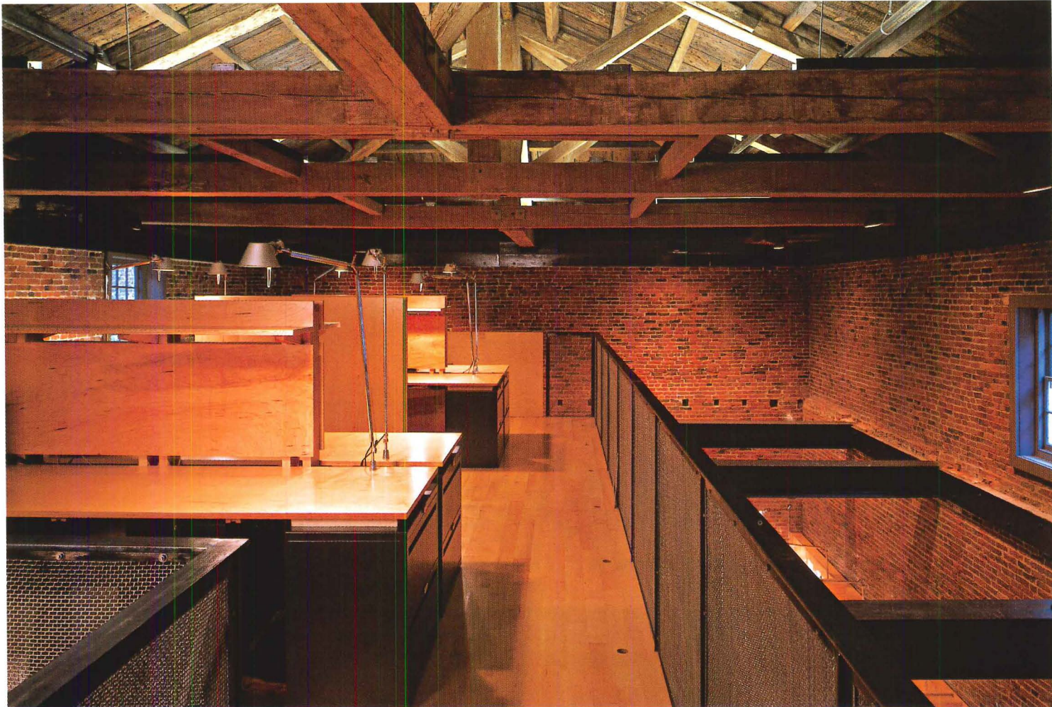
The mezzanine (above) adds nearly 500 square feet of floor space. Steel beams shore up the brick walls, which were 5 inches off square. Custom furnishings (above and below) are crafted to create a handsome interior of balanced proportions.
