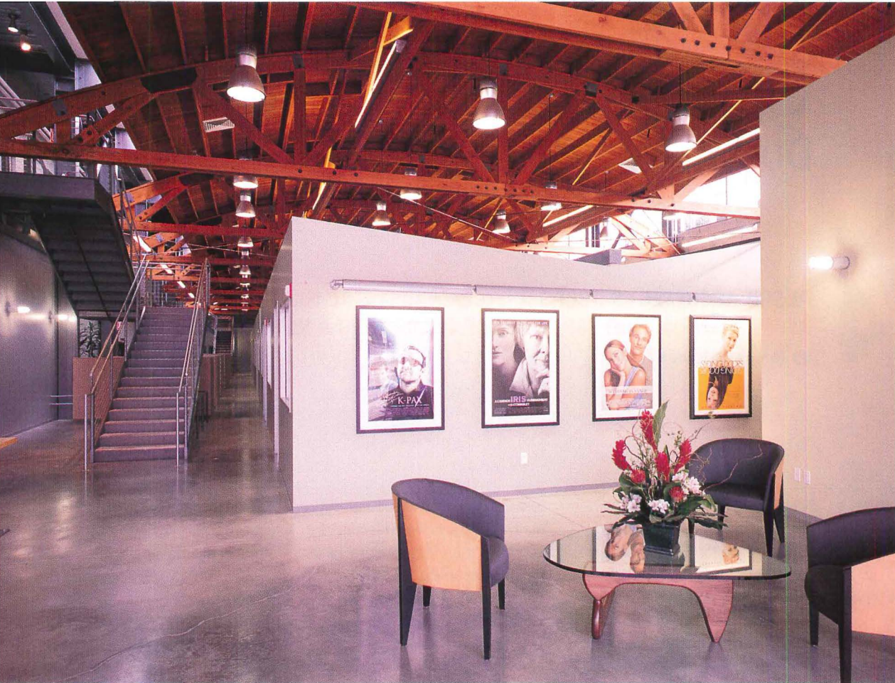
Myers added a mezzanine level to the old warehouse but kept the original bowstring trusses (left and below). A new glass tower provides vertical circulation to the office spaces (opposite).
