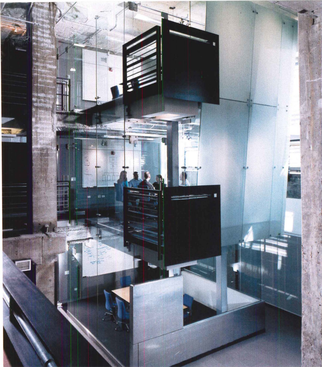
Fronted by cantilevered balconies, the glass-enclosed conference rooms are stacked in towers surrounded by open-plan offices (left). A street-level loading dock was replaced with a two-story bank of windows to infuse the below-grade floors with daylight.
