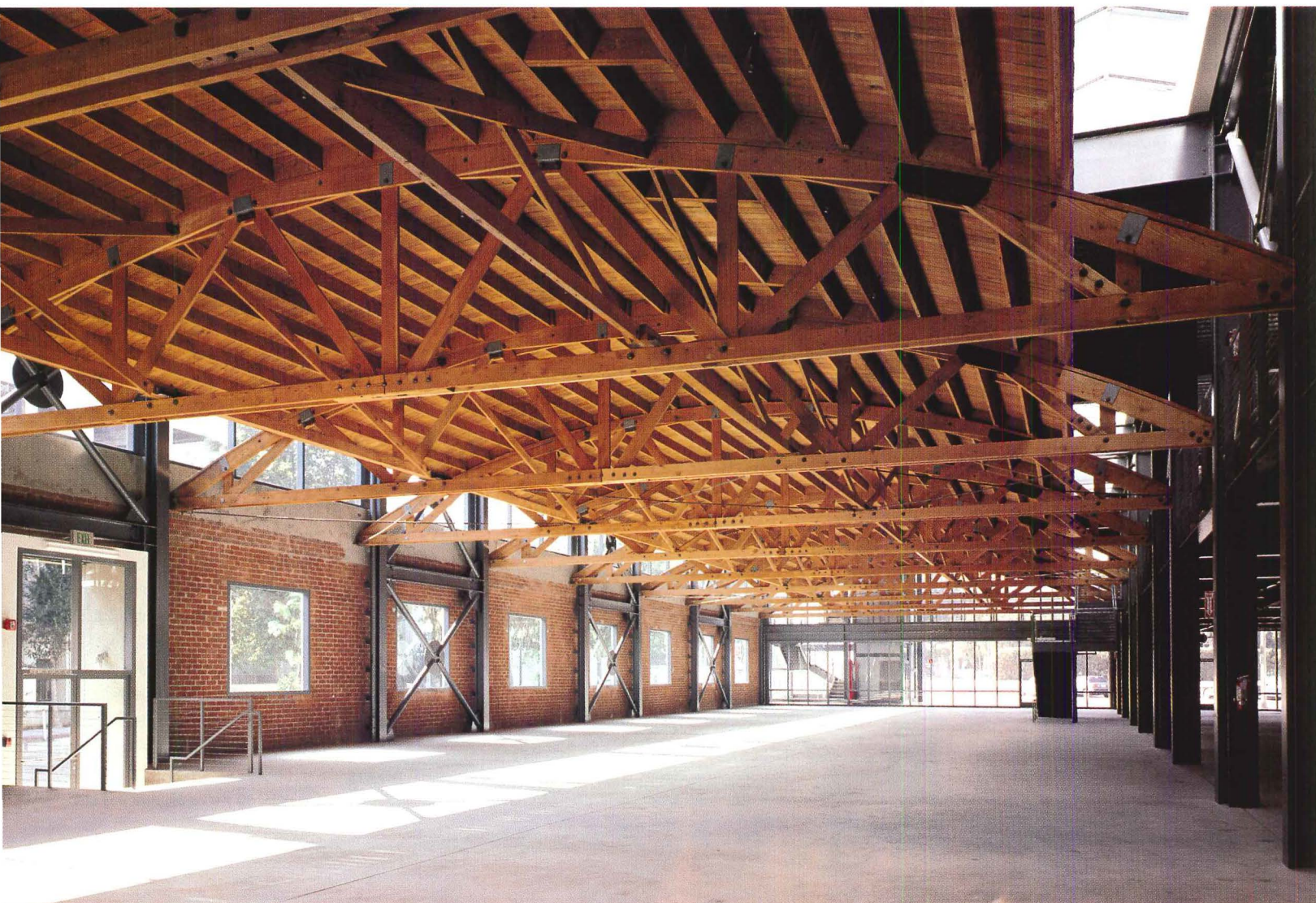
Myers added a mezzanine level to the old warehouse but kept the original bowstring trusses (left and below). A new glass tower provides vertical circulation to the office spaces (opposite).
