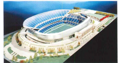
Work has begun on the Soldier Field reconstruction (top), shown in a model (above).
