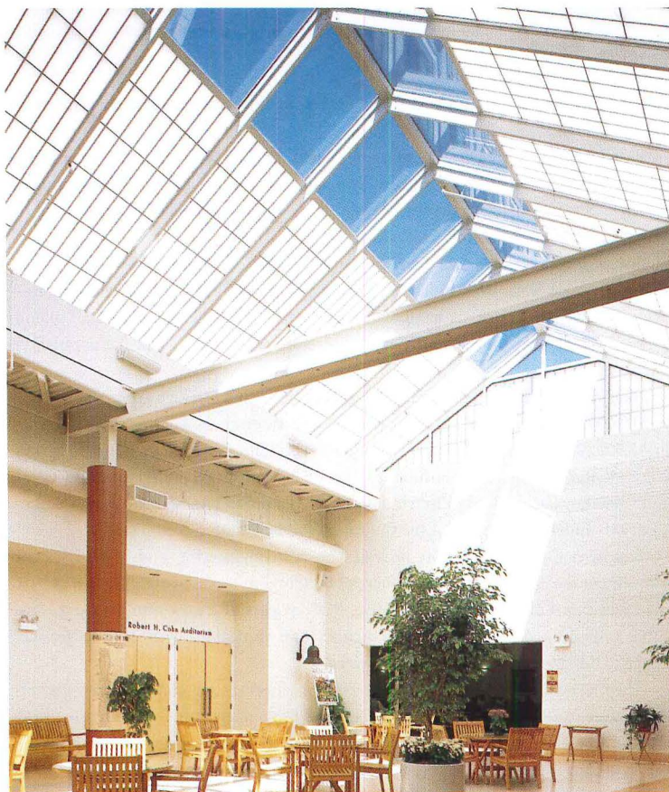
North Shore Senior Center, Northfield, IL: Skylights were added to North Shore Senior Center during recent renovation. The skylight system was installed directly over existing roof structure.
