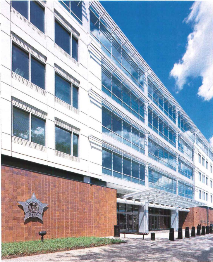
Chicago Police Headquarters, Chicago, IL To make the most efficient use of glazing systems, designers of Chicago Police Headquarters added a shading device, which is supported by the curtain wall system.
