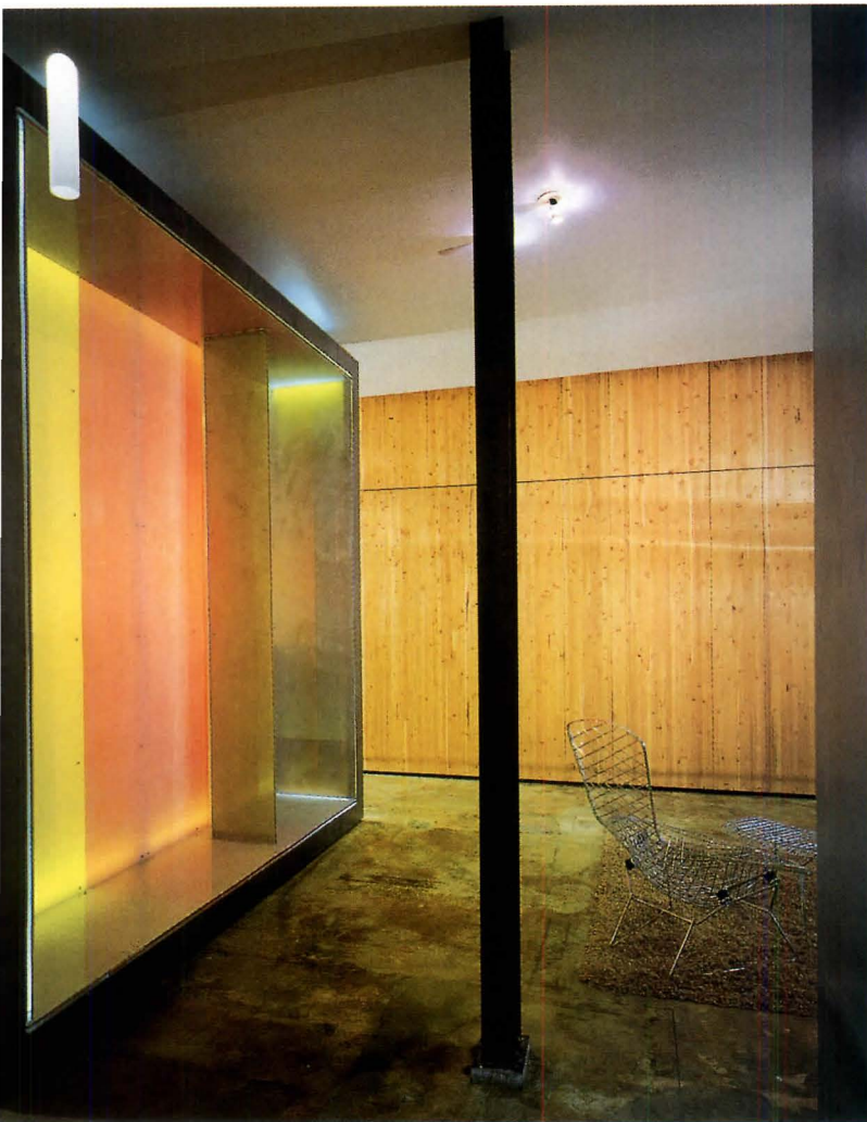
The reception desk (below) is concrete, as are the floors, which combine two different lithochrome stains.
