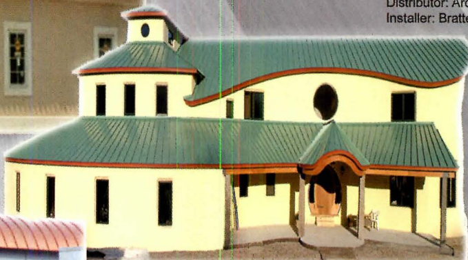
2. Residence, Freeport, ME Distributor: Cambridge Sheet Metal Co., Inc., Scarborough, ME Installer: Demmons Roofing, Inc., Portland, ME
