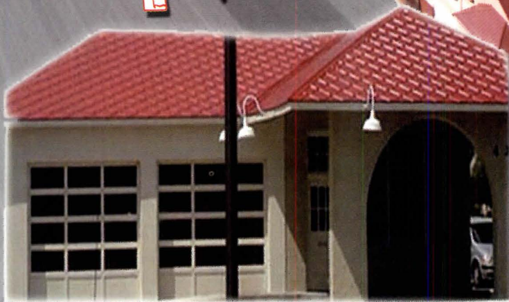
2. Kissimmee Keys Welcome Station, Kissimmee, FL Architect: Lunz Prebor Fowler Architects, Lakeland, FL Distributor: Bradco Supply Co., Tampa, FL Installer: A. Armstrong & Sons Roofing, St. Cloud, FL
