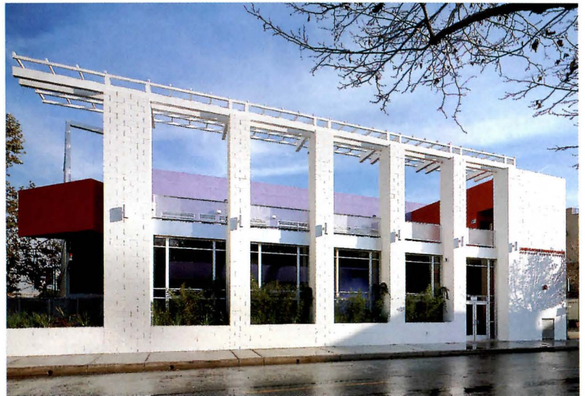
Designed by Lehrer Architects, the James M. Wood Community Center, in L.A.'s skid row, brings good design to a population that rarely has an opportunity to appreciate it.
