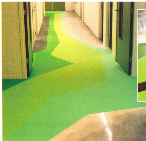
A base layer of green polyurethane was painted to give depth to the building's floor.
