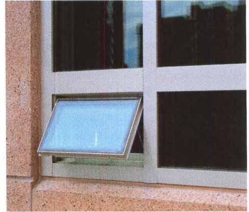
An operable vent within a curtain wall system.
