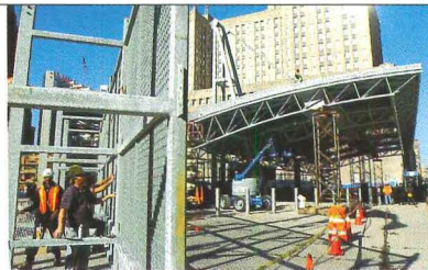
Workers completing WTC Path station.
