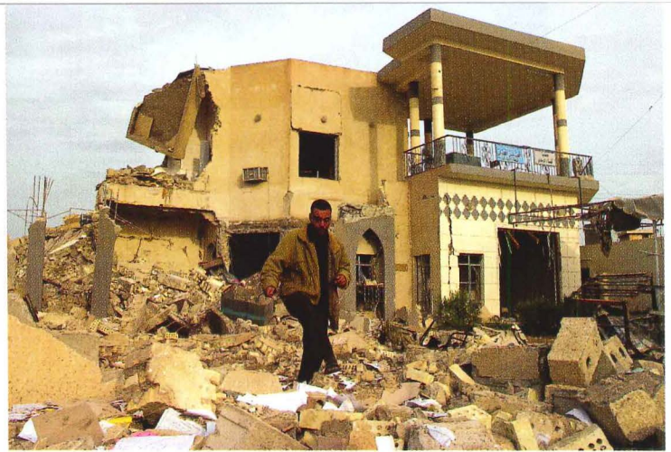
Although many buildings were destroyed during the Iraq War (above, a civic structure in Ramadi), looters are responsible for the most significant losses.
