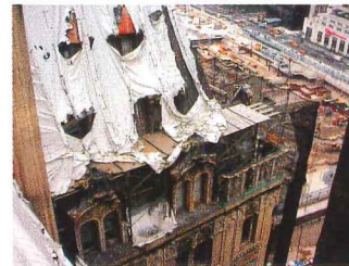
Ground Zero seen behind 90 West.
