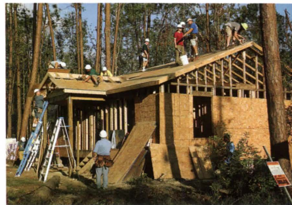
A kit-of-parts Habitat for Humanity house.
