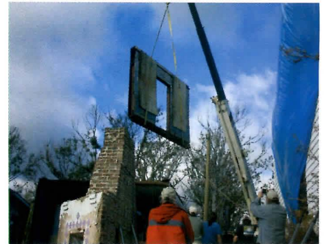
Workers dismantling the Hecker House.
