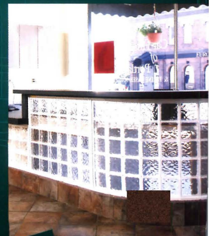
Aluminum mullins were used to connect these flat panels and radius walls together. A flat cap and mounting channel were used to mount the unit to the base and the walls. Flat caps were also used to connect the desktop to the top of the panel.
