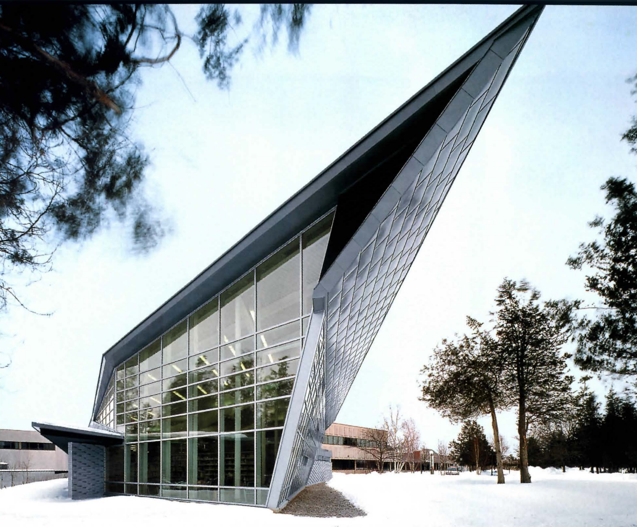
Loyalist College, Belleville, Ontario, Canada; Architect: Stephen Teeple Architects, Toronto, Ontario, Canada; Flat Lock Interlocking Wall Tiles; Fabrication and Installation: Semple Gooder, Toronto, Ontario, Canada
