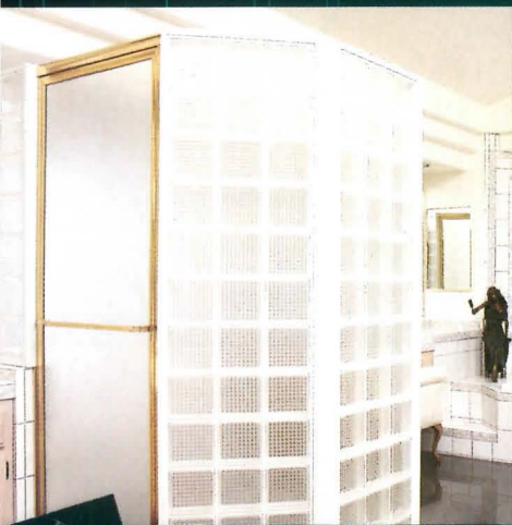
45-degree corner caps were used to connect Hy-Lite panels to form this neo-angle shower. Flat caps were used to finish off the top and sides of the doorway, while a flat cap and mounting channel were used to attach the panels to the curb and wall.
