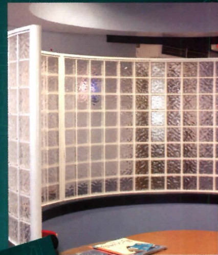
Round caps finished off the ends of this radius wall perfectly. Aluminum mullins were used to connect the three radius walls together, while a flat cap mounted the units to the top of the curved wall.
