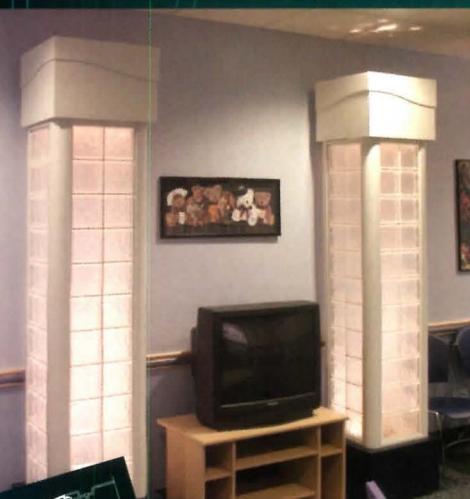
90-degree corner caps were used to connect four acrylic block panels together to form decorative, lit towers. The panels were mounted to the base and top piece with flat caps.
