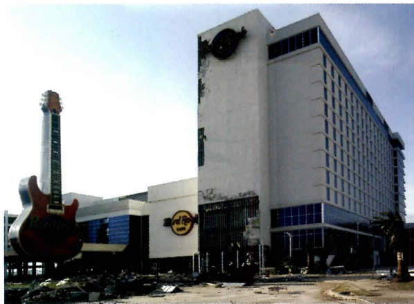
The Hard Rock Casino in Biloxi, Mississippi, was badly damaged by Hurricane Katrina.
