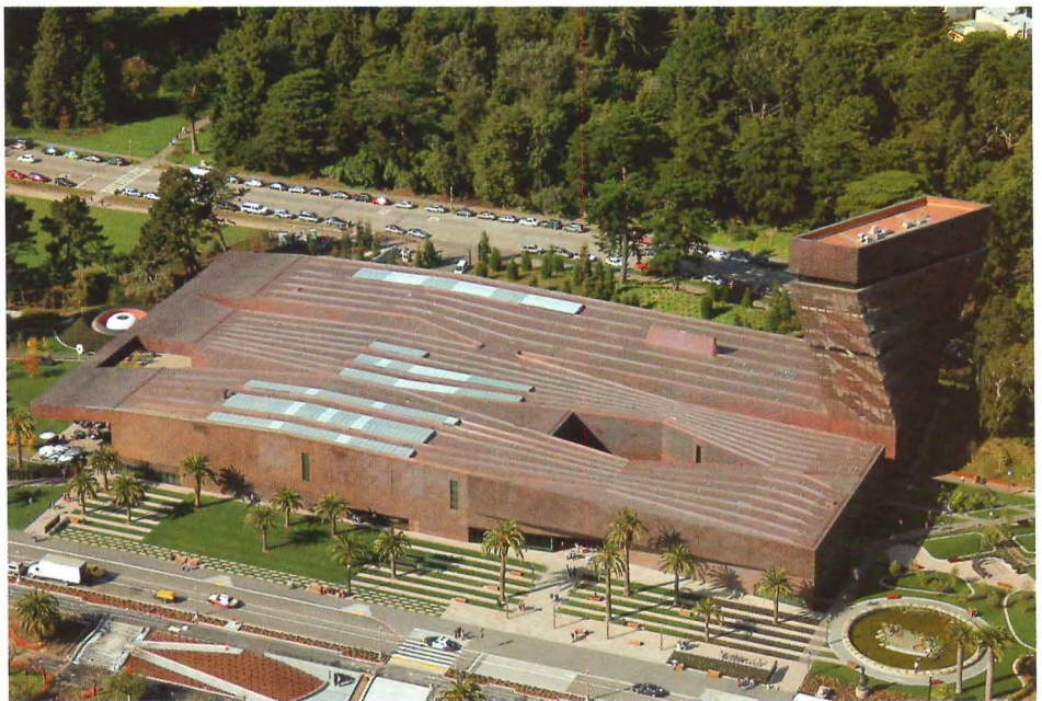
Contiguous but separate structures make up the de Young. The galleries occupy a three-story building interwoven with courtyards, and a 144-foot-tall twisting tower houses educational programs.
