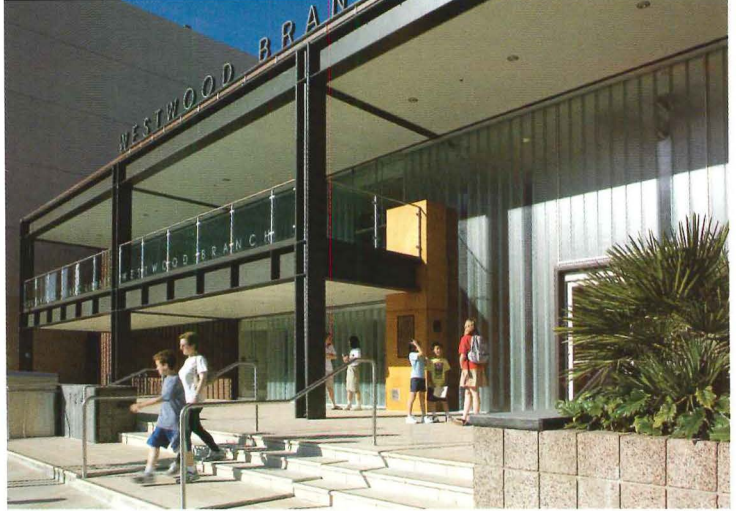
Channel glass in the facade of Steven Ehrlich Architects' Westwood Branch, in L.A., controls light levels and blocks views of parking lots across the street.
