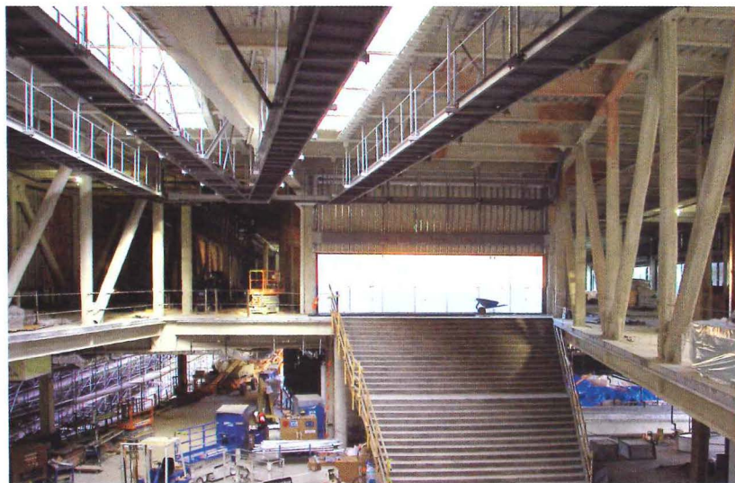
The owner’s desire for a museum with as many large, column-free spaces as possible resulted in long spans, one more than 90 feet, and trusses as deep as 20 feet.
