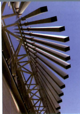
Eskew+Dumez+Ripple's "wave wall" (left) is composed of 122 pivoting aluminum tubes arrayed across the LIGO Science Education Center, in Livingston, Louisiana. Wayne Troyer Architect won a Merit Award for its own studio, inside a converted New Orleans warehouse (below left).
