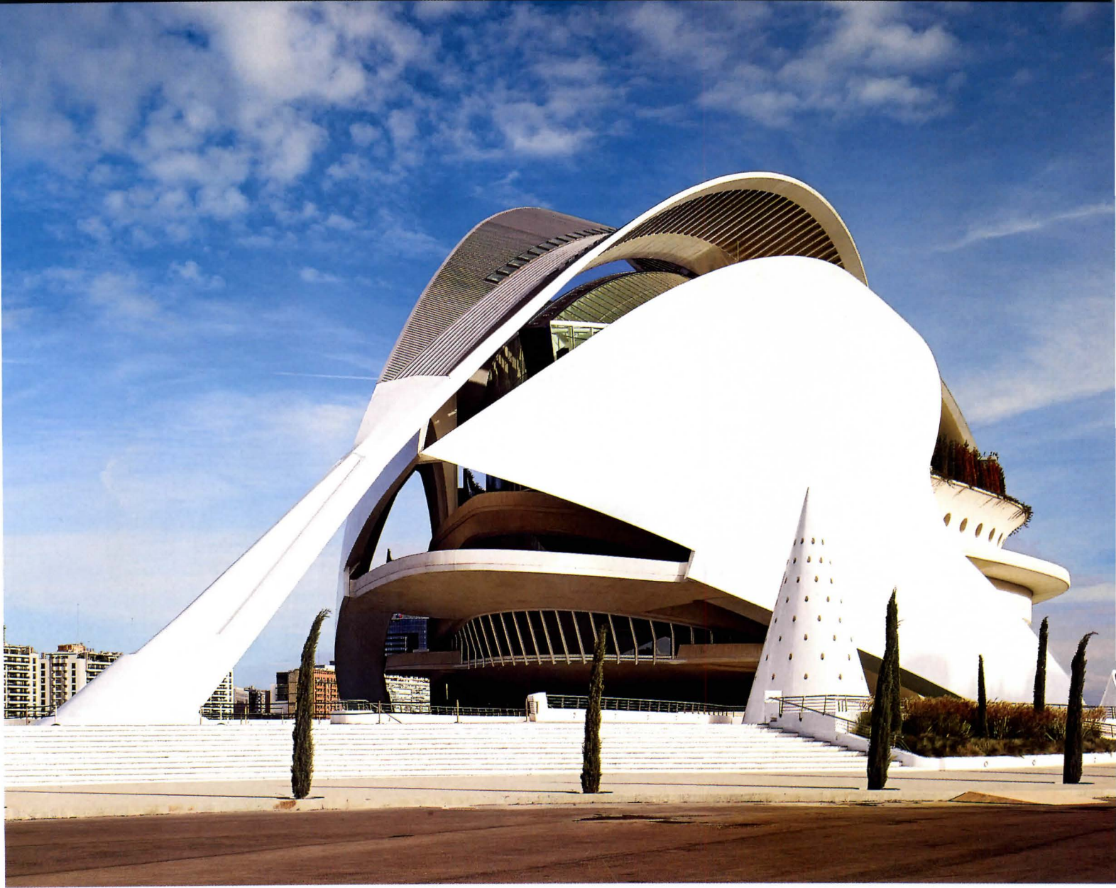
Perforated cones beside the opera house (above) house elevators that connect the street and plaza levels. The Hemispheric Planetarium/IMAX theater evokes a human eyeball, socket, and lid—all set over a vast reflecting pool (right). East of the planetarium, right beside the water, is the longitudinal Prince Felipe Science Museum (at far right in photo, right).
