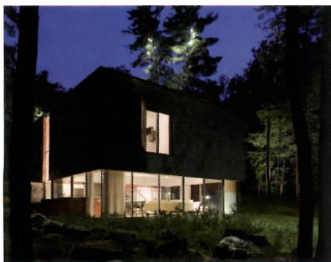
Gluck designed the guest units as inverted twins with a transparent living/dining space on the lower floor of one (left) and the top of the other (bottom). Each unit has its own set of stairs (below).
