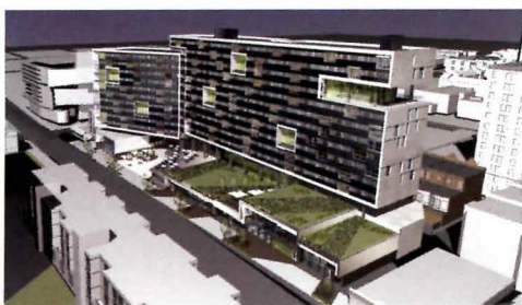
A green roof will cap the Radian's street-level shops.
