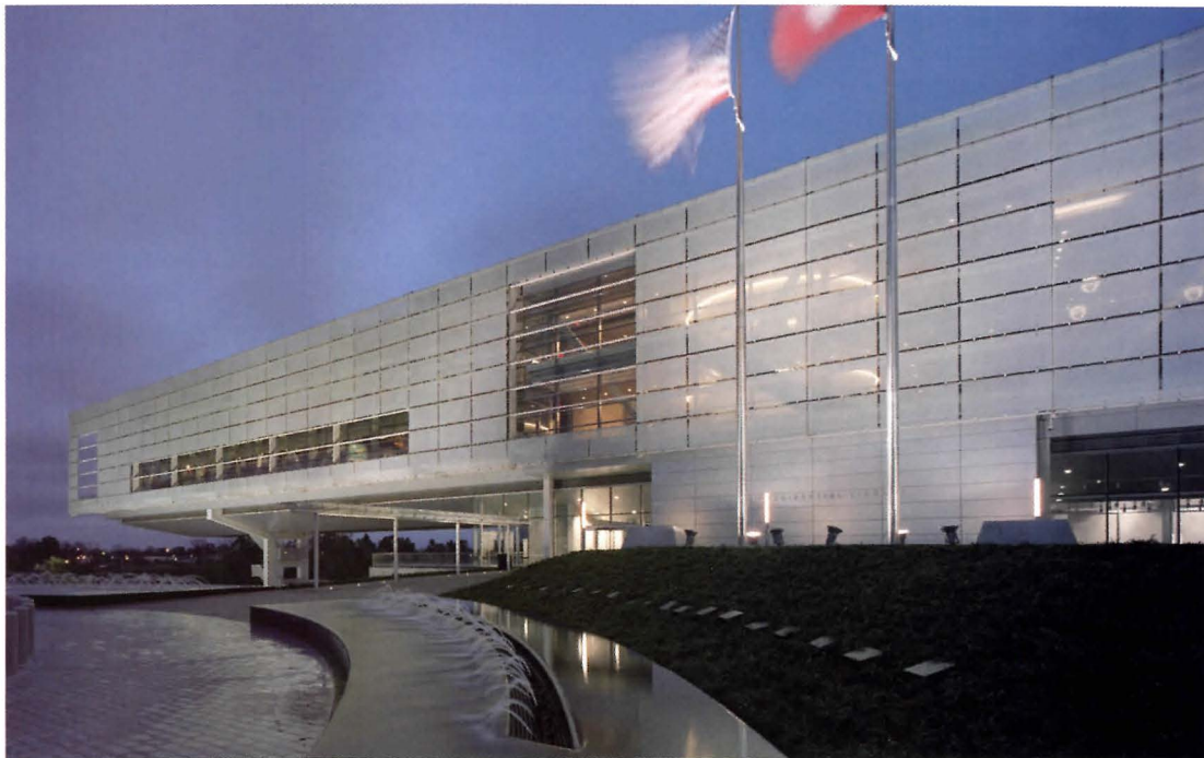
Two previously certified NC projects, the Clinton Library (above) and the Solaire (right), are seeking EB certification at the Platinum level.
