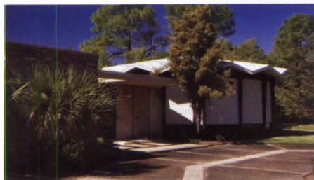
The Cohen residence, shortly before demolition.
