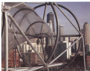
The wind turbines on the top of Near North in Chicago (page 147).
