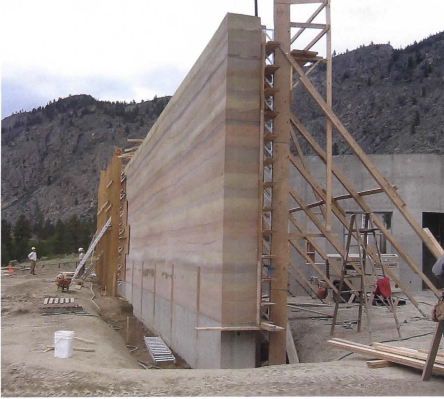
A rendering (below) illustrates the scope of the project. Formwork for rammed-earth construction is similar to that of concrete, although construction is more time consuming (above).
