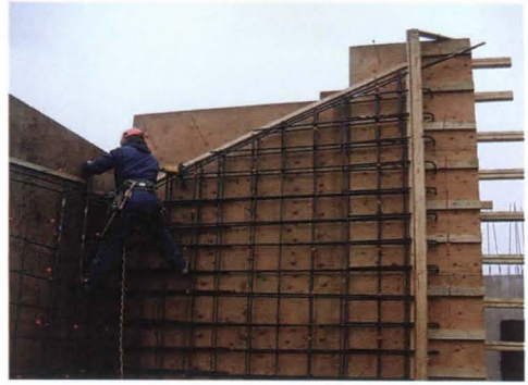
The contractors say rammed-earth walls such as this one will withstand a 3,500-psi water stream.
