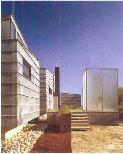
An outdoor shower (left) sits adjacent to the house's main entrance, acting as a beacon at night. A fire pit (below) is made of the same concrete block used for the house's foundation.
