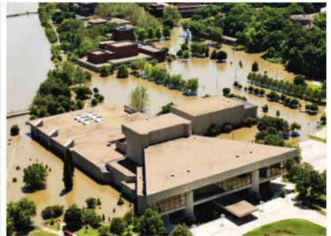
Hancher Auditorium was heavily damaged by the 2008 flood.
