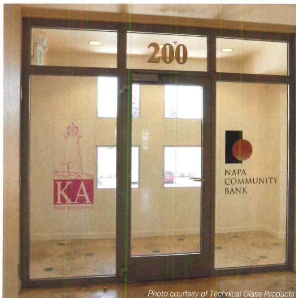
Depending on the product, fire-rated glazing can be etched on one side without affecting its fire-rating.
