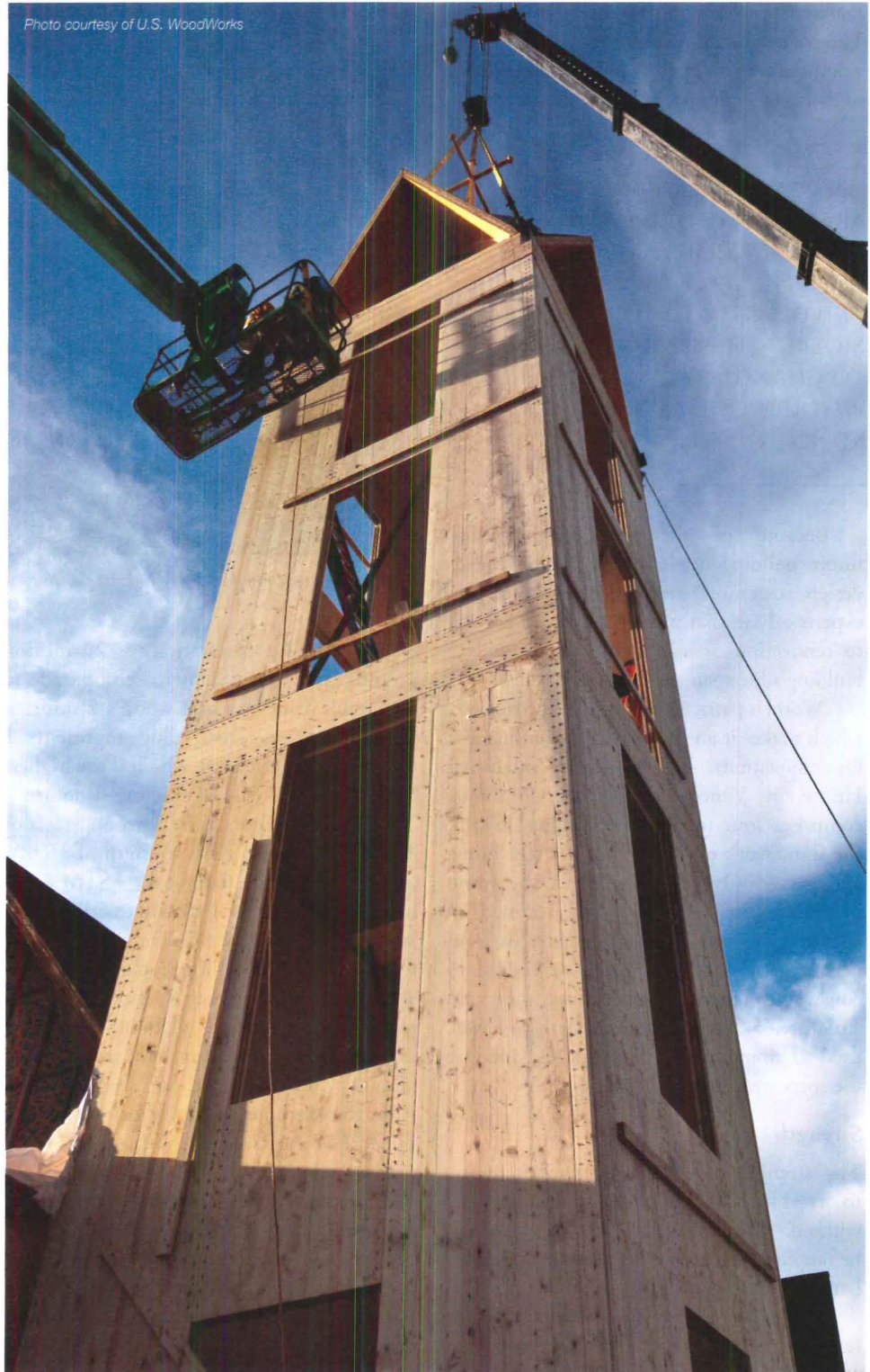
A 78-foot bell tower at Myers Memorial United Methodist Church in Gastonia, North Carolina is the first non-residential structure in the U.S. to be built from cross laminated timber.
