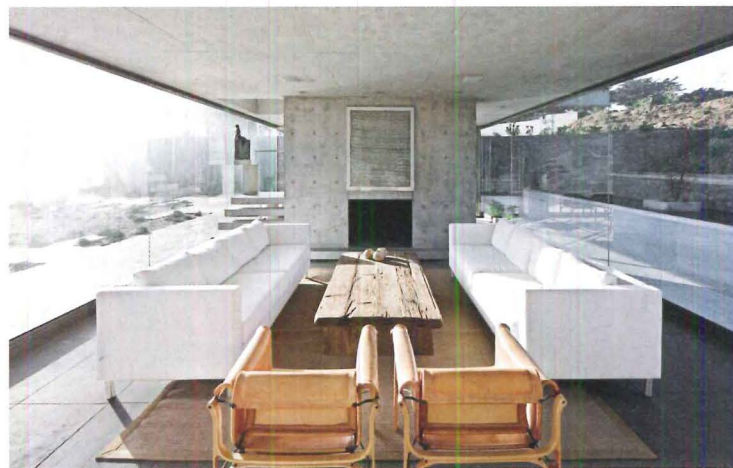
CENTER: Long post-tensioned, reinforced-concrete beams cantilevered at the ends shield second-level sitting areas and bedrooms of the houses.
