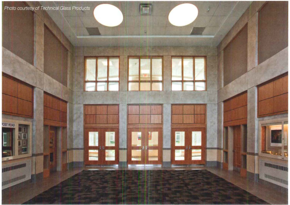
This school has a mix of different fire-rated ceramic glazing units.
