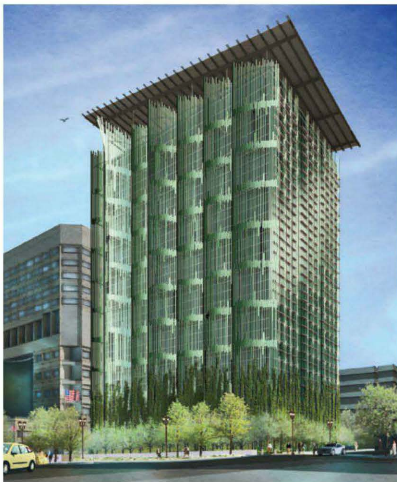
LACY VEIL The $133 million renovation of the 1970s Edith Green/Wendell Wyatt Federal Building (far left), in Portland, Oregon, includes installation of a high-performance glass skin shaded by a system of aluminum "reeds" (left).
