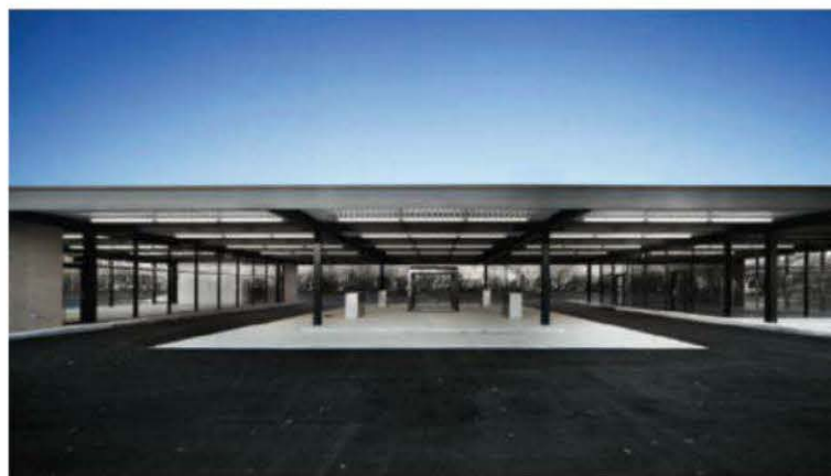
TOP: Located in the Czech Republic, the Villa Tugendhat (1930) was named a UNESCO World Heritage Site in 2001. ABOVE: A Mies-designed gas station in Montreal is now a community center for youths and seniors.
