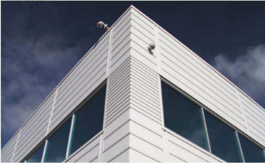
ICBPs are based on metal exterior panel and rainscreen design principles.
