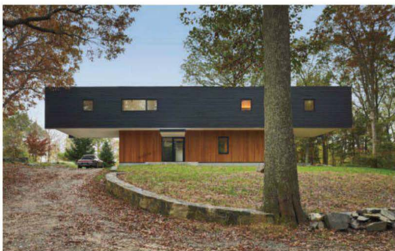
HANGING OUT Large window walls maximize views and daylight for the main living spaces on the second floor (above). Clad in black-stained cedar, the upper story cantilevers 20 feet from each end (right). Polished concrete floors contain a radiant-heating system in the south-facing living room (below).
