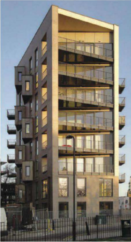
When it was constructed in 2011, Bridport House was the largest timber-built apartment block in the world.
