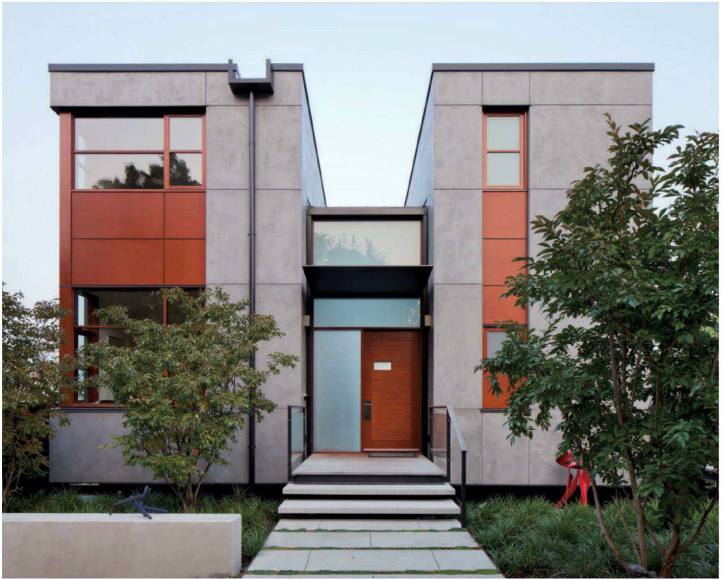
Capitol Hill / Balance Associates / Seattle, W.A. / Application: External / Product: Facade / Finish: Copper
