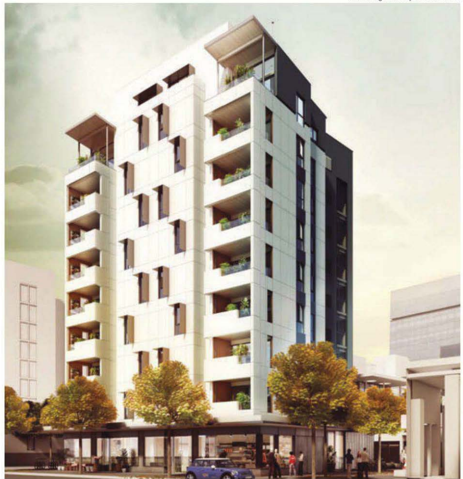
At 10 stories tall, Forté in Melbourne, Australia, was the tallest timber apartment in the world when it was completed in 2012.
