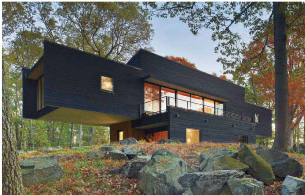
HANGING OUT Large window walls maximize views and daylight for the main living spaces on the second floor (above). Clad in black-stained cedar, the upper story cantilevers 20 feet from each end (right). Polished concrete floors contain a radiant-heating system in the south-facing living room (below).
