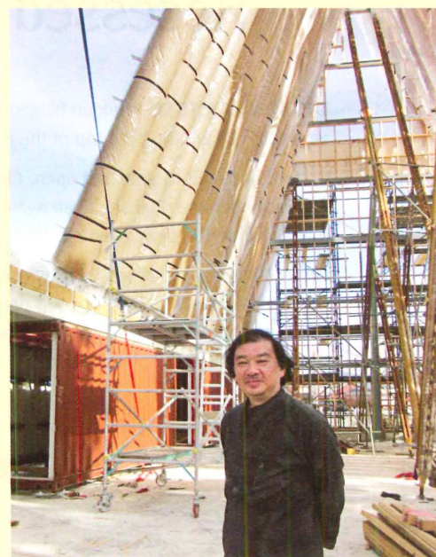
Shigeru Ban in front of his cardboard cathedral. The roof will rise up to 70 feet above the altar.
