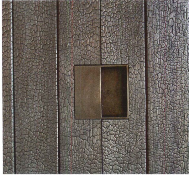
BURN THIS A door has a custom pull that works for both lefties and righties; Caleb Coy chars Spanish cedar.
