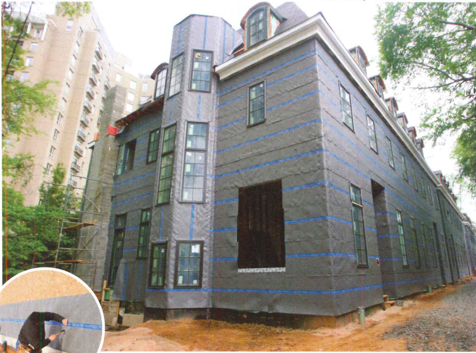
A ventilated rainscreen over a polymeric, water-resistive barrier protects the enclosure for Bellingrath Town Residences in Atlanta's Buckhead.
