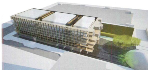
Cubiform offices on the perimeter wrap around white laboratory volumes separated by the atriums.
