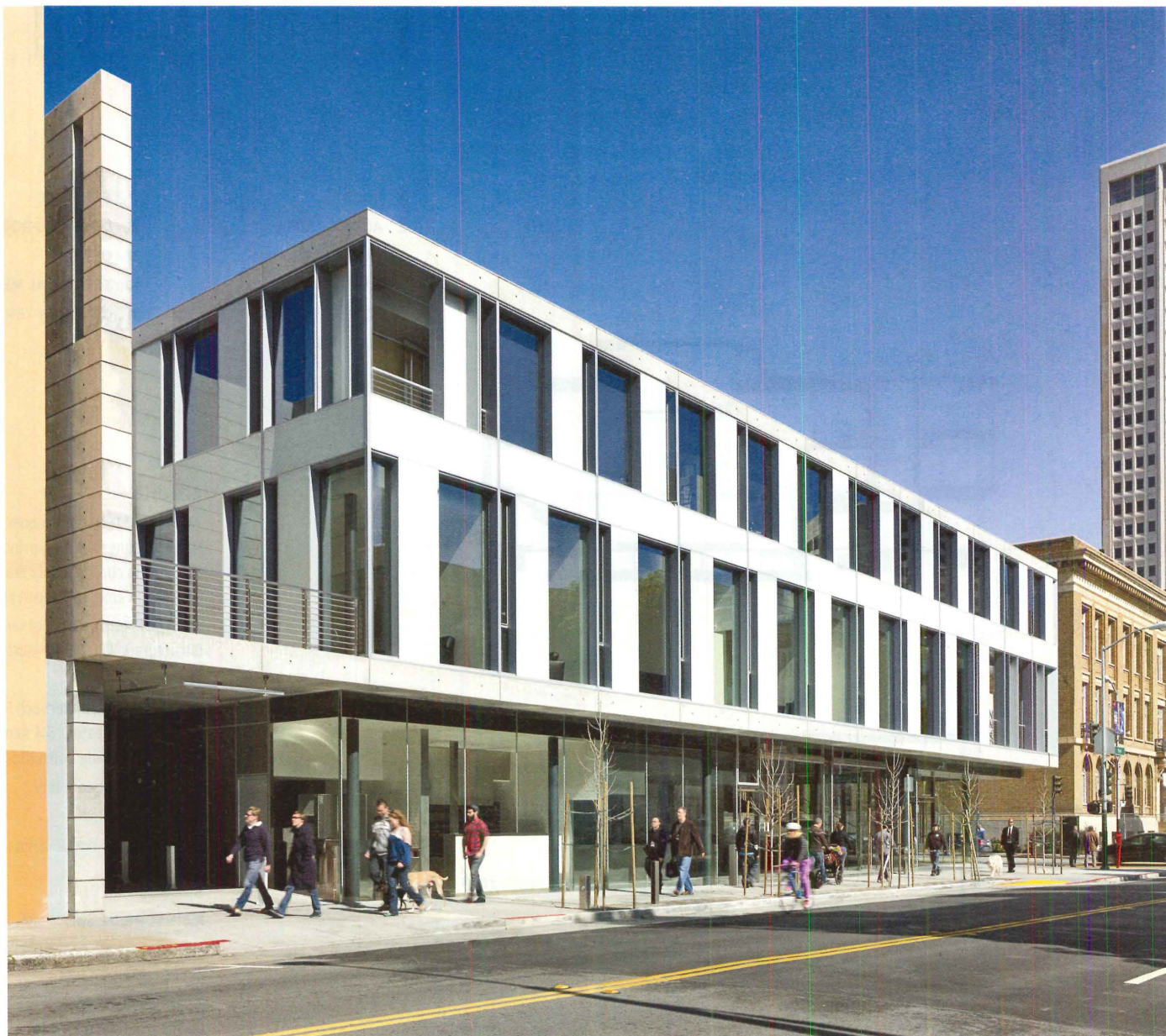
DISCREET TRANSPARENCY The architects pierced the poured-in-place-concrete structure with glass window walls so pedestrians standing outside the south facade (right) or the north facade (opposite) can observe activities within.
