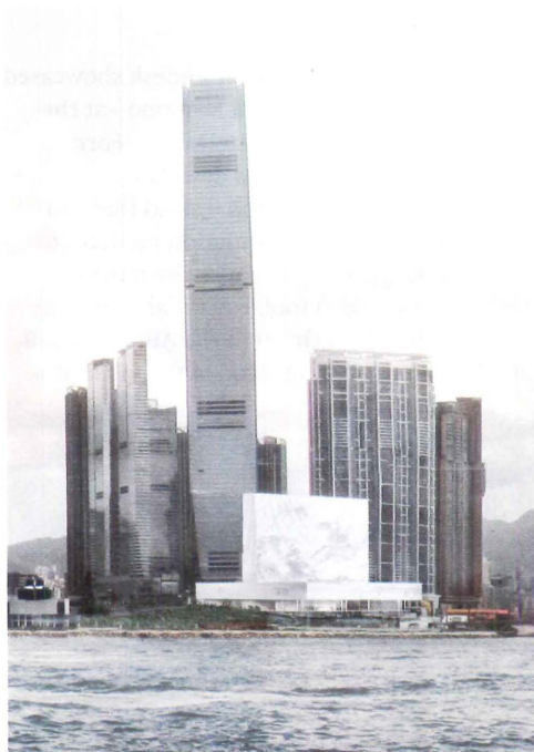
The upside-down-T-shaped museum is planned for a site in front of KPF's International Commerce Centre tower.
