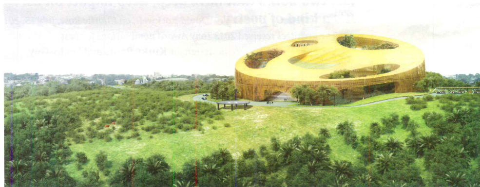
Auditoriums, conference spaces, and dining facilities are organized around three garden courtyards, which are linked by an interior promenade. The angled roof collects rainwater that is then recycled for use in the building.
